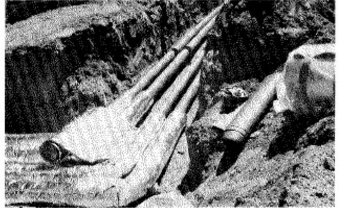
Pipe elbows shown wrapped in double wraps of foil faced fiberglass insulation. Straight lengths of wax coated corrugated cardboard piping are shown at right of photo.
